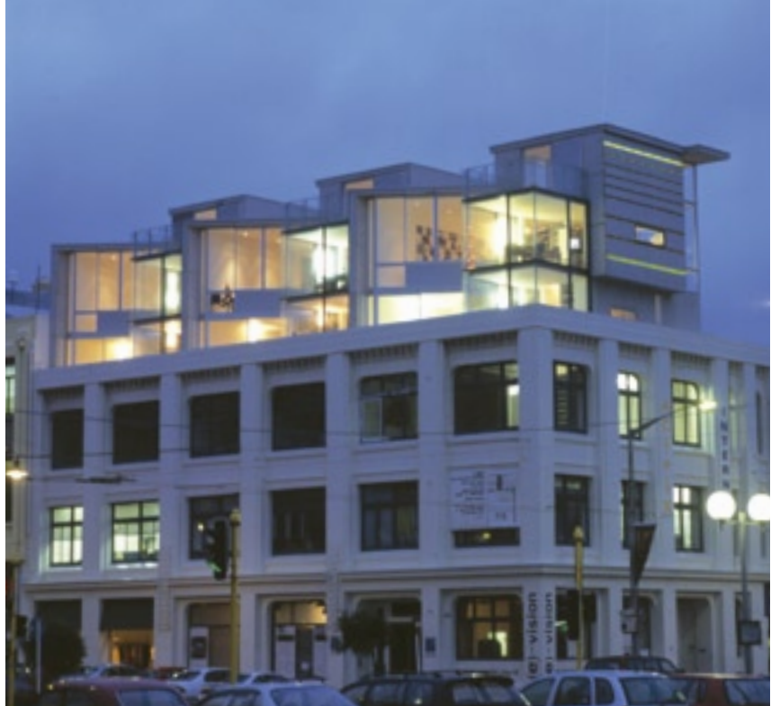
Adaptive reuse with new residential maisonettes on the upper levels above three floors of retail and commercial.
