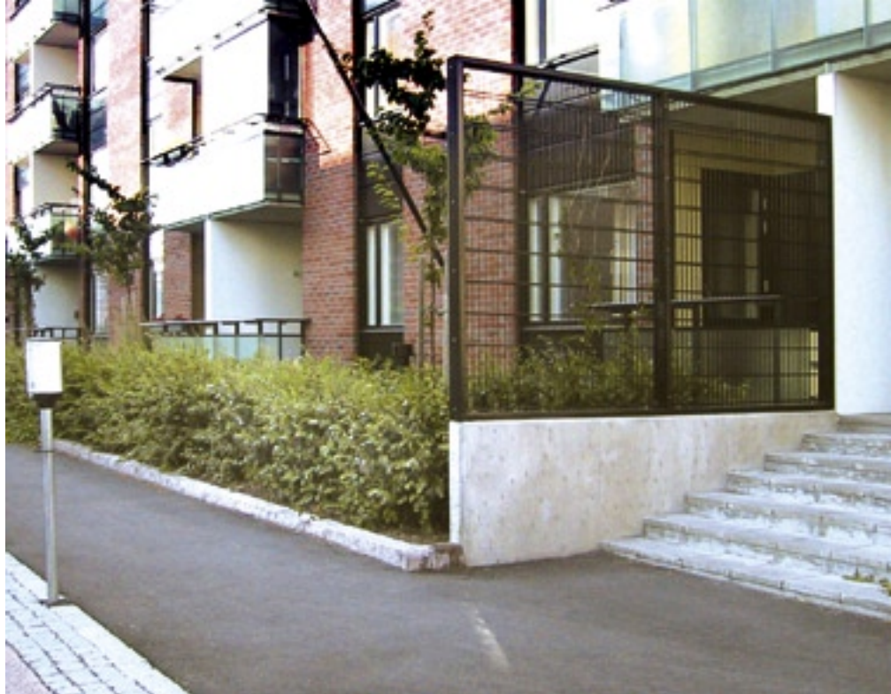
Planting will soon grow over the screen to provide added privacy for the ground floor apartment from the building entrance area. The garden provides added separation from the public footpath.
