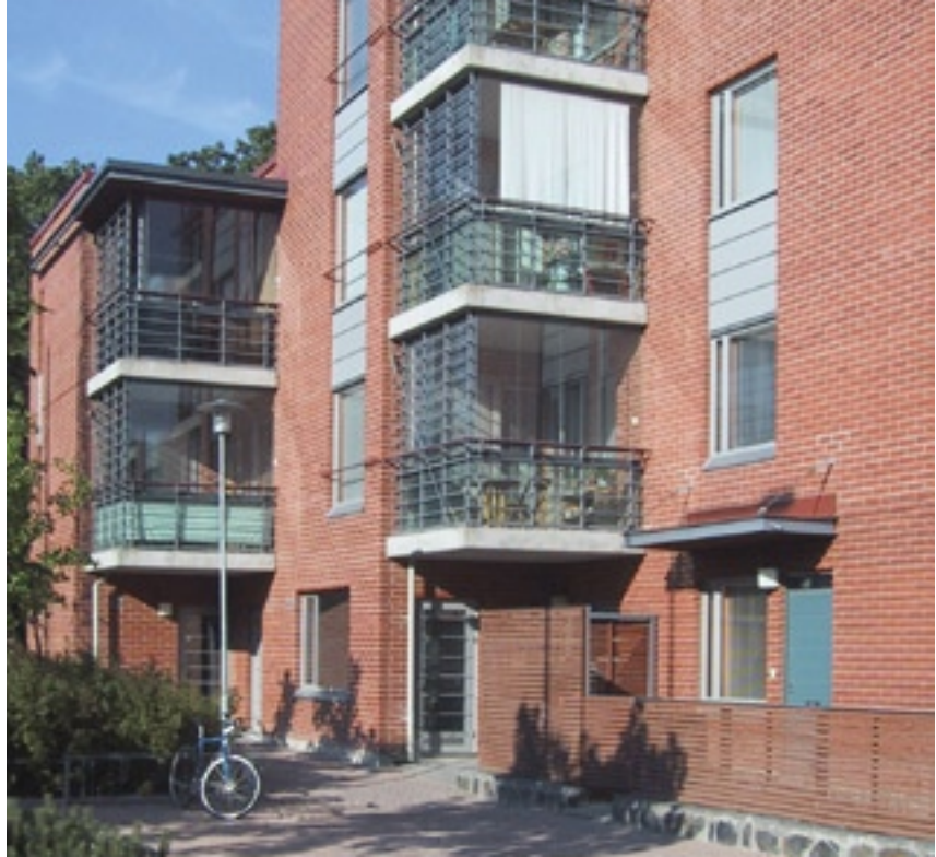
The use of folding glazed panels and high-mass structure allows these balconies to act as heat stores in colder months.
