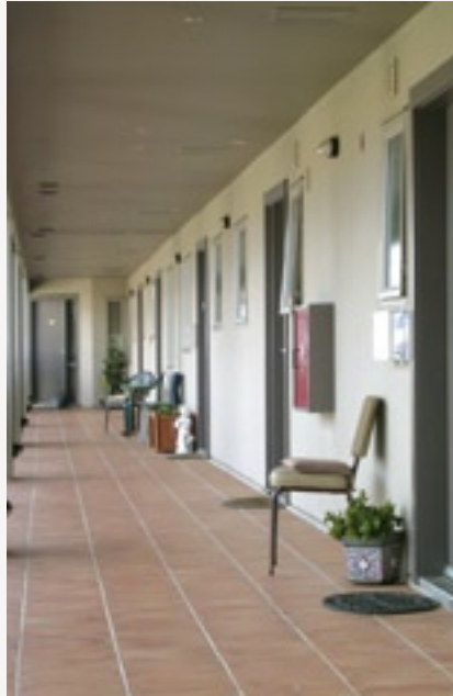
The width of the west-facing horizontal access balconies allows a degree of occupation by residents.
