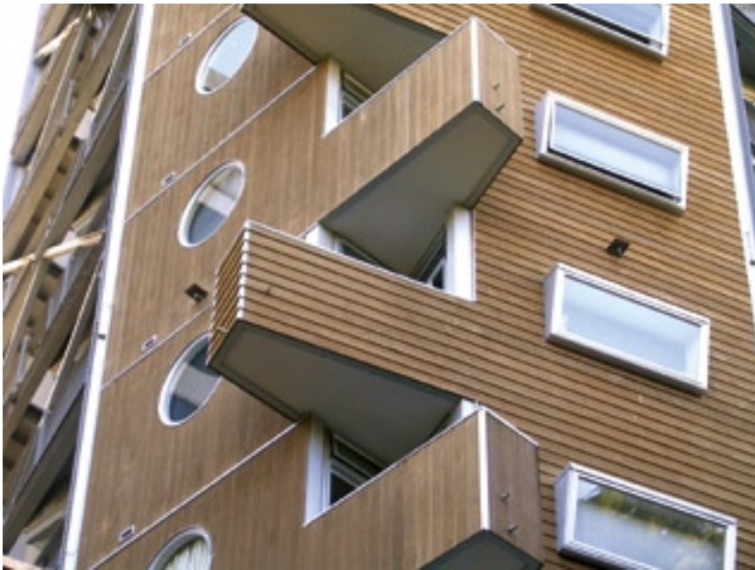
Junctions, especially between dissimilar materials, require a commitment to careful detailing.
