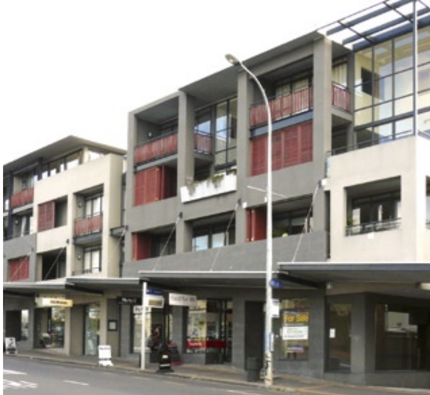
Double height glazing on the upper levels of this development allow daylight to reach well back into a deep plan.
