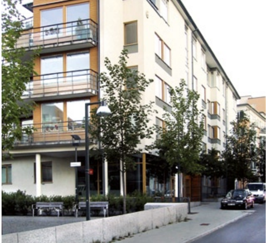
An outdoor area with good lighting and well overlooked by apartments.
