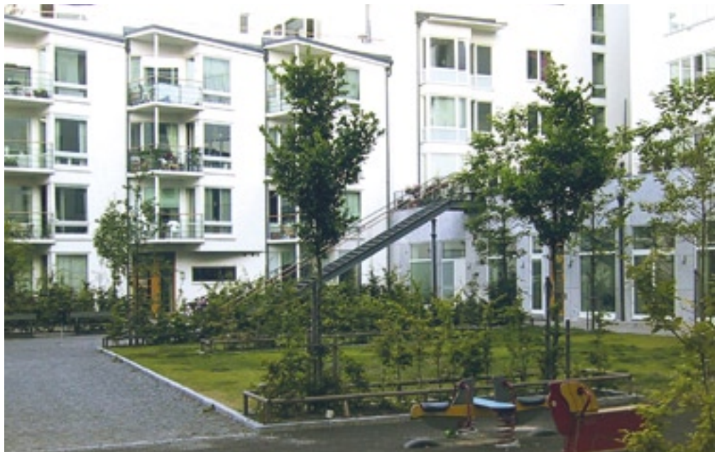
Communal open space including children's play area connects via stairs to another communal area above.
