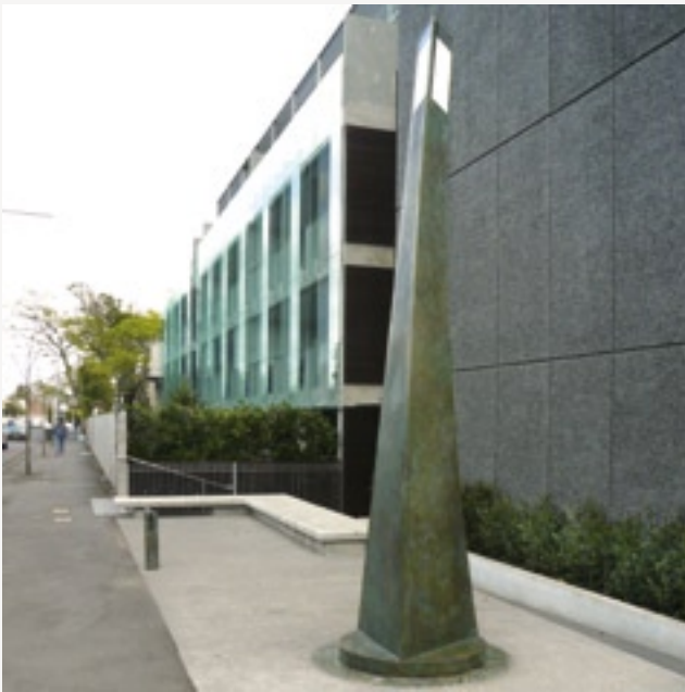
Site corner has been given over to public open space, including an artwork. This adds identity to the development & emphasises the main entry.
