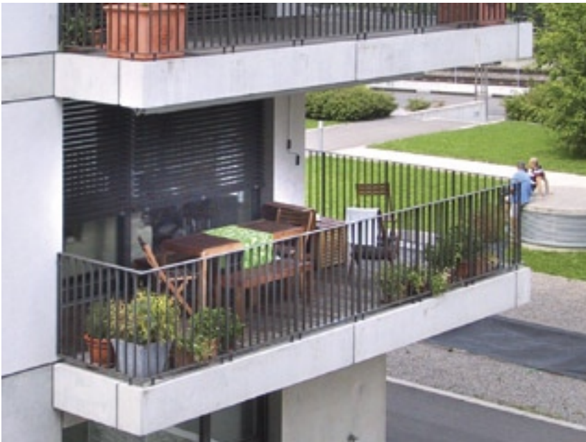
A semi-recessed balcony that overlooks communal open space.
