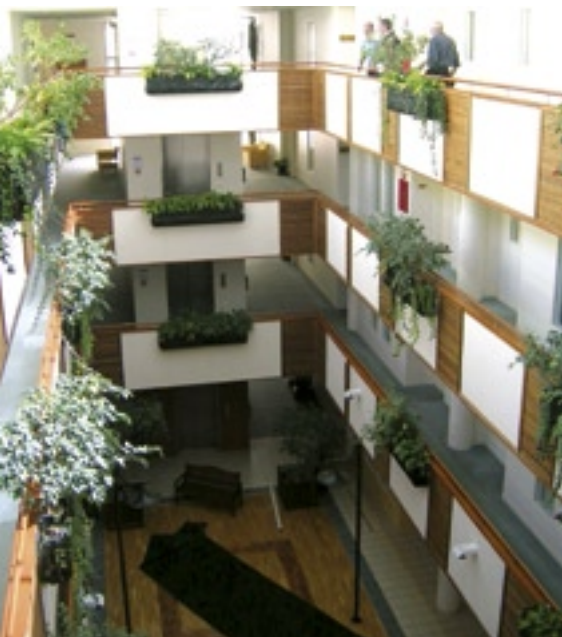
Atrium provides natural light to accessways and communal recreation space at ground floor.
