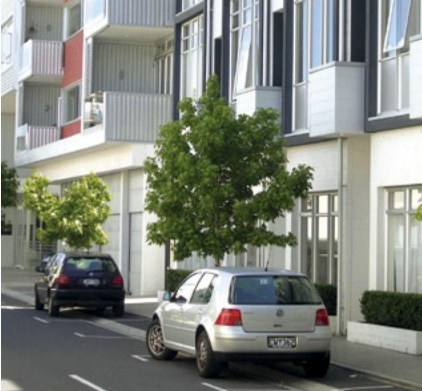
Bay windows and balconies help provide better casual surveillance of the street.
