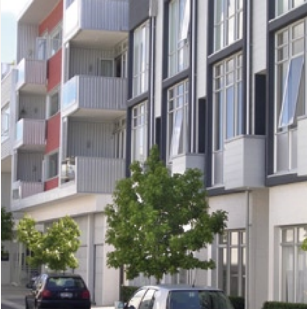
Terrace housing (foreground) beside a four-storey apartment block.
