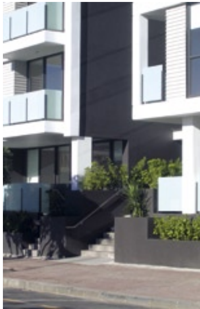
A change in level, hedge and non-transparent glass balustrades all contribute to retention of privacy for these ground floor apartments.
