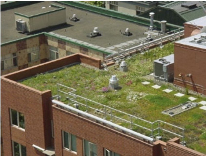
Green roofs can reduce and filter stormwater discharge from the site while providing additional amenity for residents.
