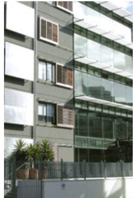
External fixtures are used here to provide both sun protection and privacy.
