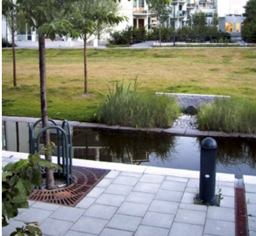
Stormwater reticulation incorporated into landscape design.
