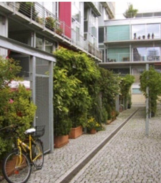
The fence to the left has been designed to allow separation of private open space from a communal courtyard. Most occupants have used vegetation grown on the fence to give the required amount of privacy.
