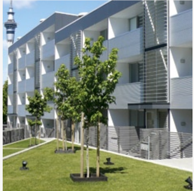
Stage 3 apartment blocks. Privacy measures for ground floor private open spaces are not particularly effective.
