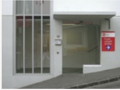
Far left: A public car park is contained within lower levels of the building.
