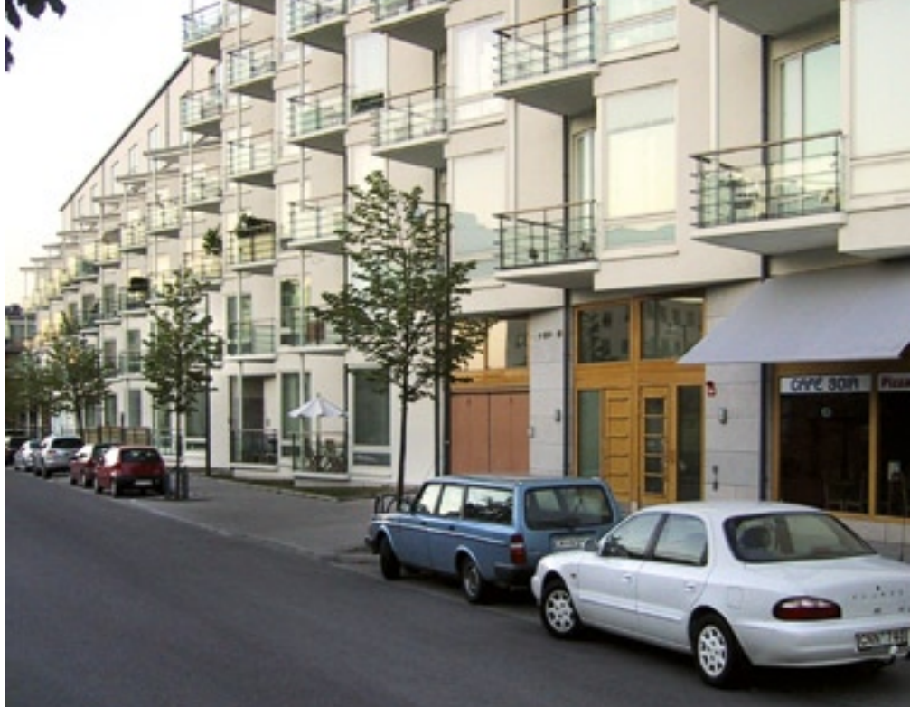
High floor-to-floor heights on the ground floor of this apartment development allow for commercial uses.
