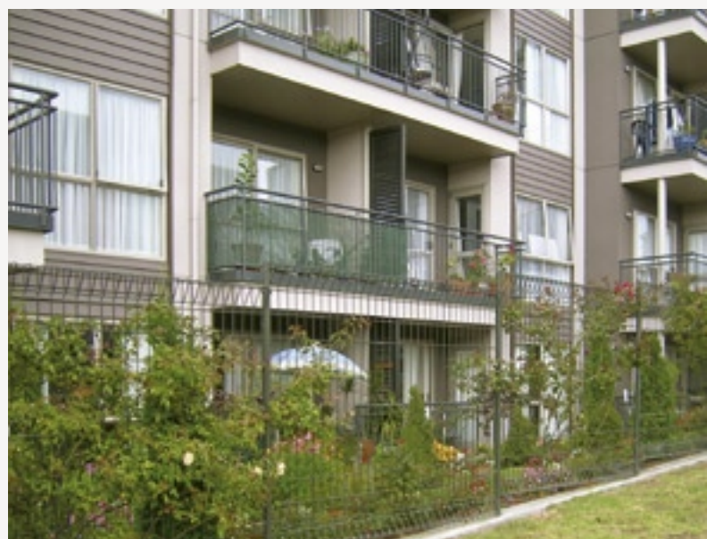
Three- and four-storey blocks have varied and articulated facades.
