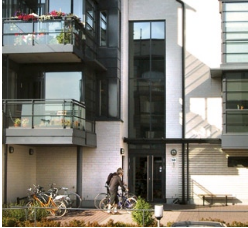
Vertical access here serves four corner aspect apartments on each floor.
