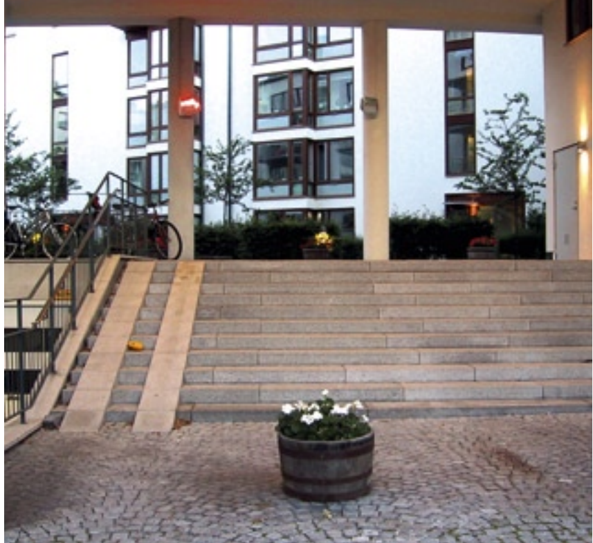
Ramps allow bicycles and prams to be pushed up and down stairs more easily.
