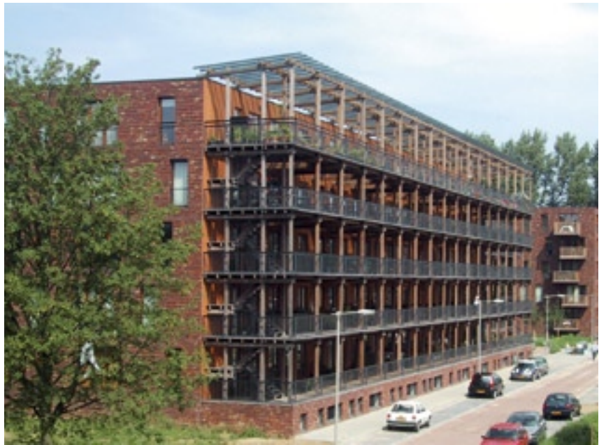
These horizontal access decks have been pulled away from the building face to give extra privacy and light to this side of dual aspect apartments.
