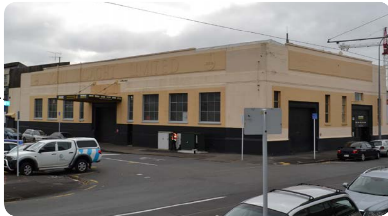
127 Pakenham Street Built Circa 1940's Previously Southern Spars (Carbon Fibre) Now North Sails New Zealand Ltd
