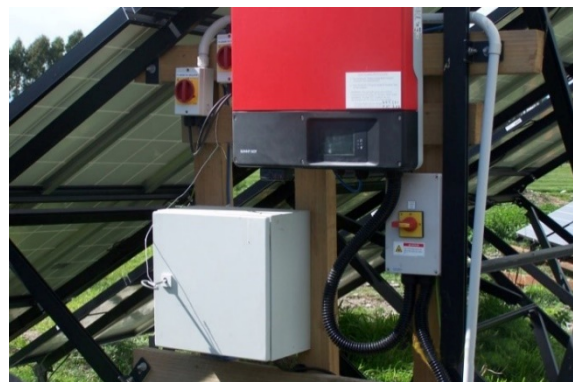
Fixed polycrystalline installations and a grid tied inverter system.
