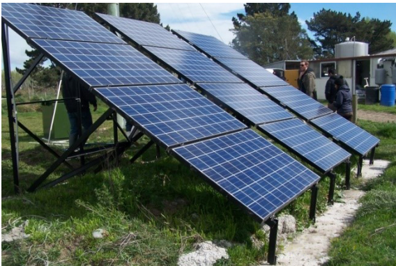
Fixed polycrystalline installations and a grid tied inverter system.
