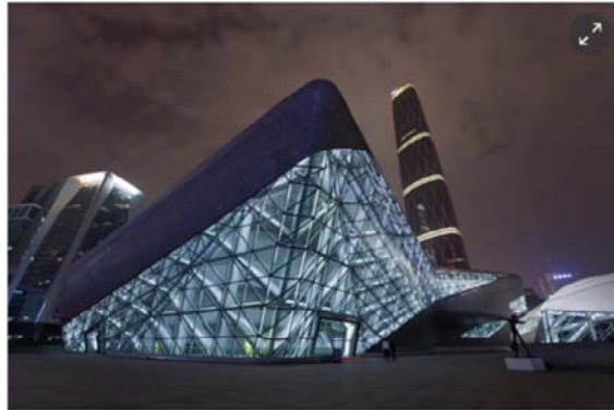
Guangzhou opera house, China. Photograph: Dan Chung for the Guardian
